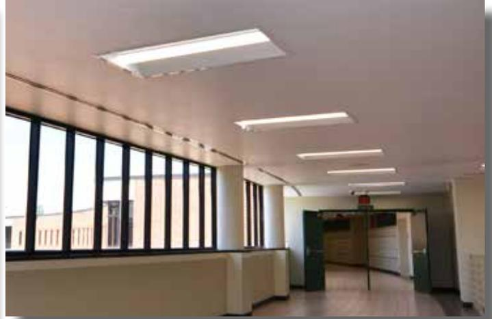
**ACR:** A recessed luminaire designed to provide diffused illumination, eliminate glare and provide a significant reduction in energy cost
